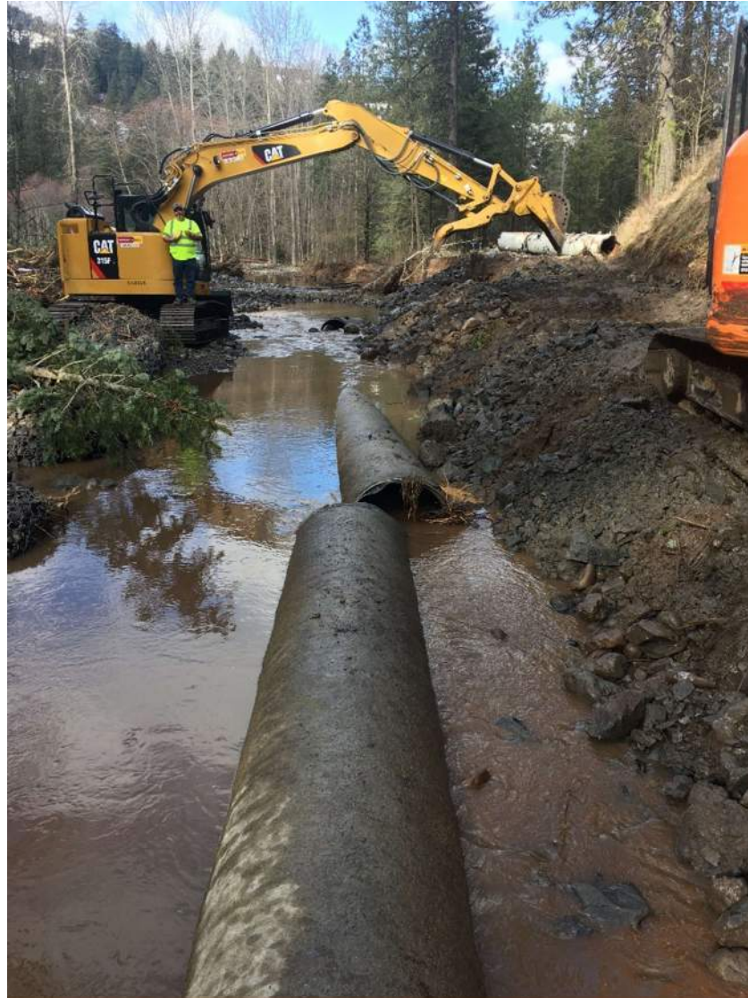
PHOTO ABOVE – UPSTREAM END OF WASHOUT 1 SEVERED PIPE
