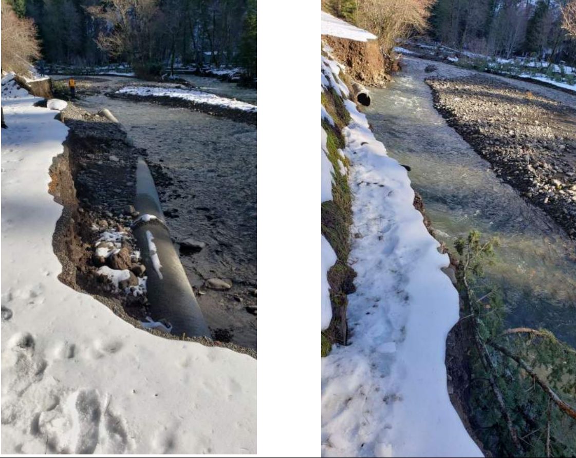
Figure 3-3. Site#3 – Upper. Looking upstream at damaged & missing pipe segments.
