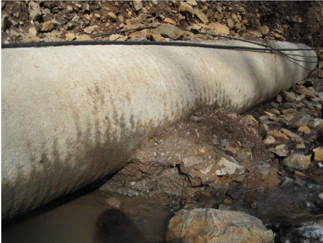
Figure 2-4. Undermined section of exposed pipe in Site #2.
