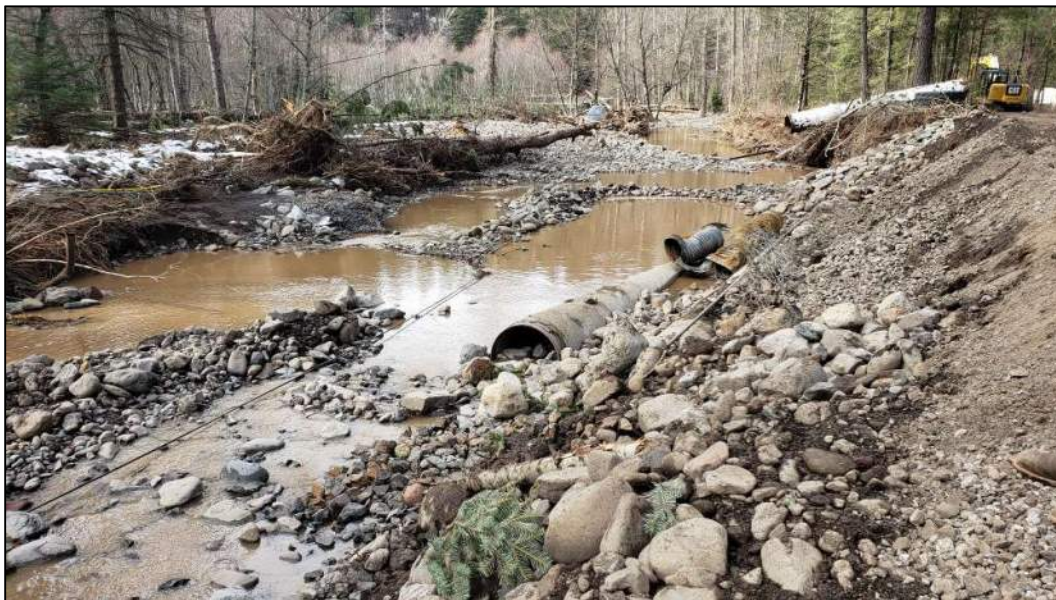
Figure 1-5. Site #1 looking downstream at damaged water transmission line.
