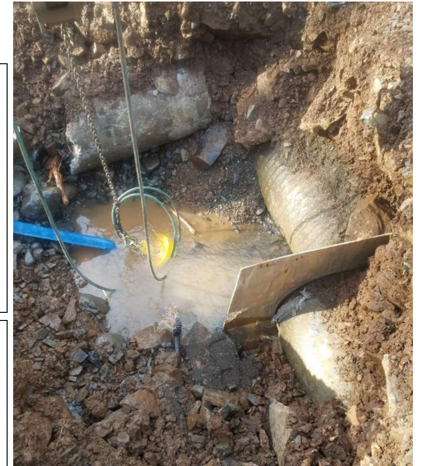
PHOTO ABOVE – UPSTREAM END OF WASHOUT 1 SEVERED PIPE PHOTO BELOW – CURRENT CONDITIONS OF WASHOUT 1
