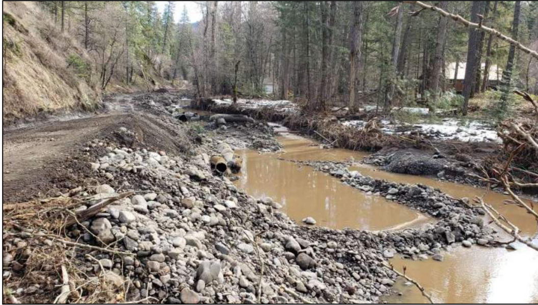
Figure 1-4. Site #1 looking upstream at damaged water transmission line.
